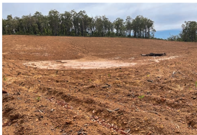
Early stage rehabilitation.
